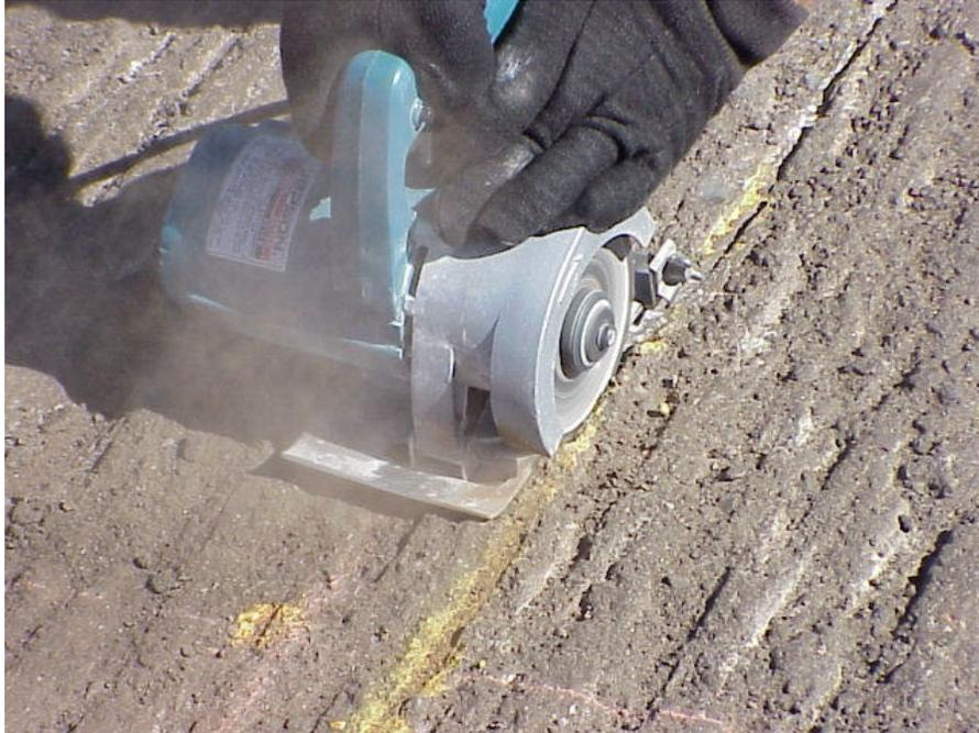
(a) Cutting groove using a diamond grinder
