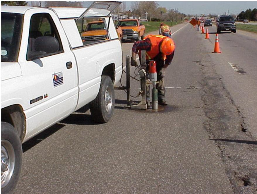
**FIGURE 5. CORING ON EXISTING ASPHALT PAVEMENT**
