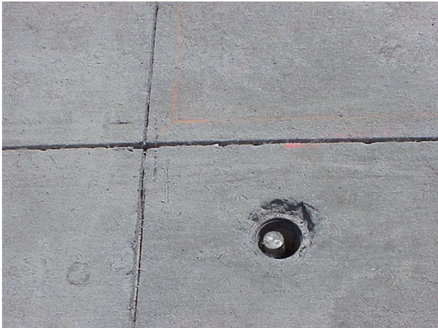
**Figure 39. A Reference Rod After Concrete Paving**
