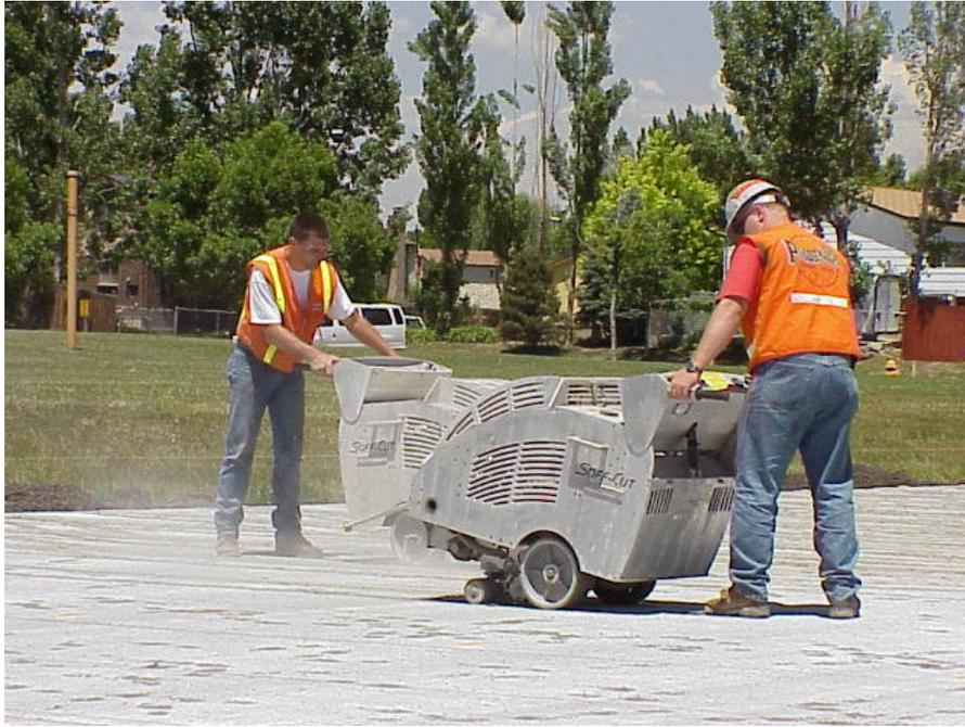
**Figure 36. Sawing Transverse Control Joints**
