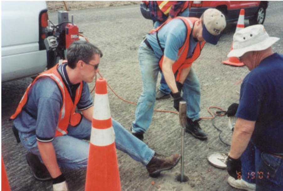
**Figure 16. Installation of Reference Rods**
