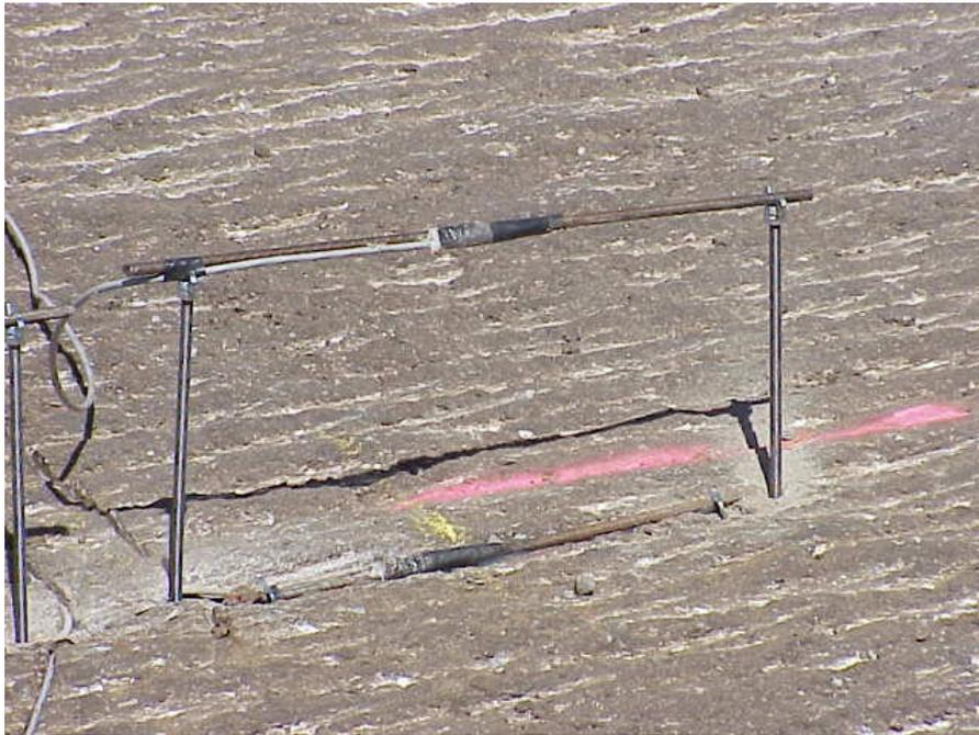
**Figure 13. Installation of Embedded Strain Gages**
