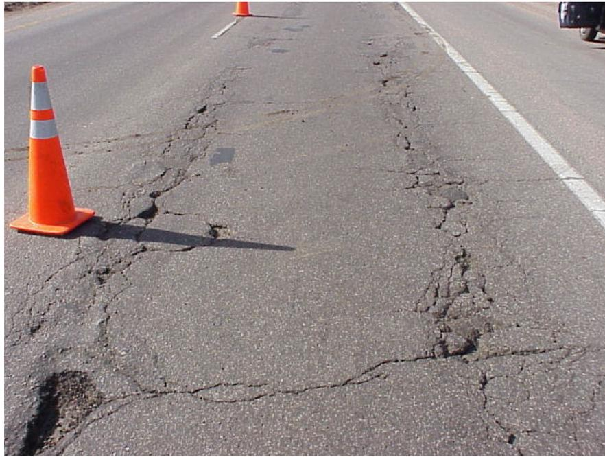
**FIGURE 2. FATIGUE CRACKING OF TEST SECTIONS 1 AND 2**
