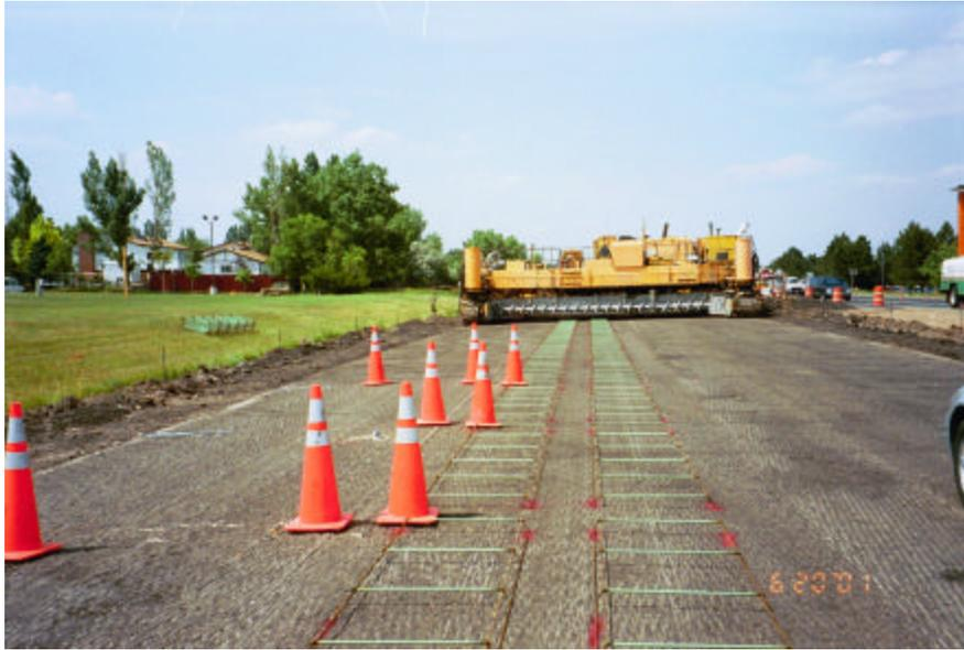
**Figure 33. Tie Bar Assembly for Test Section 1**
