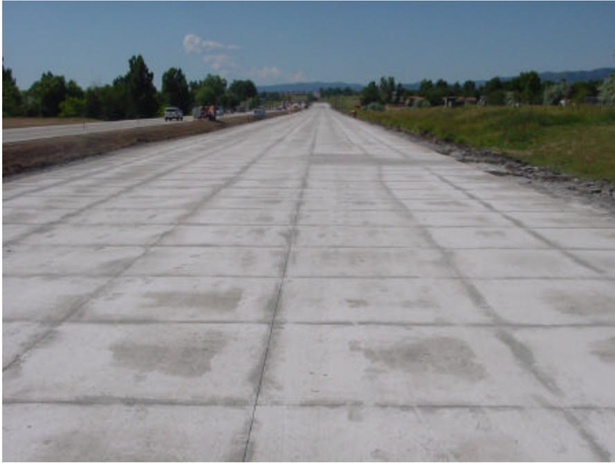
**Figure 38. Pavement Surface After Joint Sawing**
