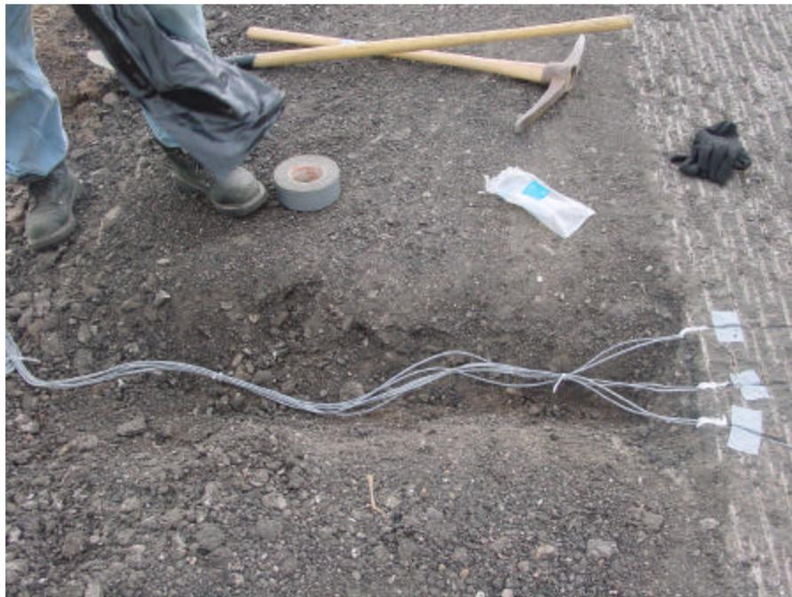
**Figure 15. Recess and Protection of Lead Wires**
