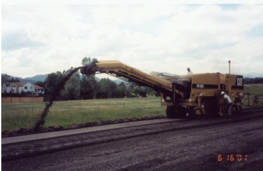
**Figure 30. Milling of Existing Asphalt Pavement**
