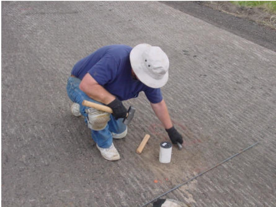
**Figure 18. Completed Reference Rod Installation**
