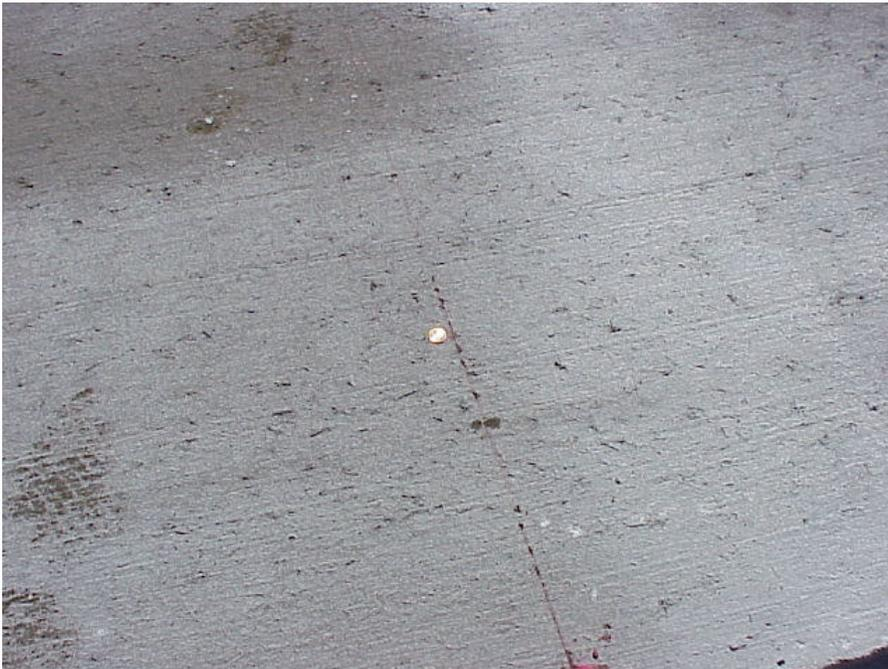
**Figure 35. Surface Texture Provided by Astro turf Drag**
