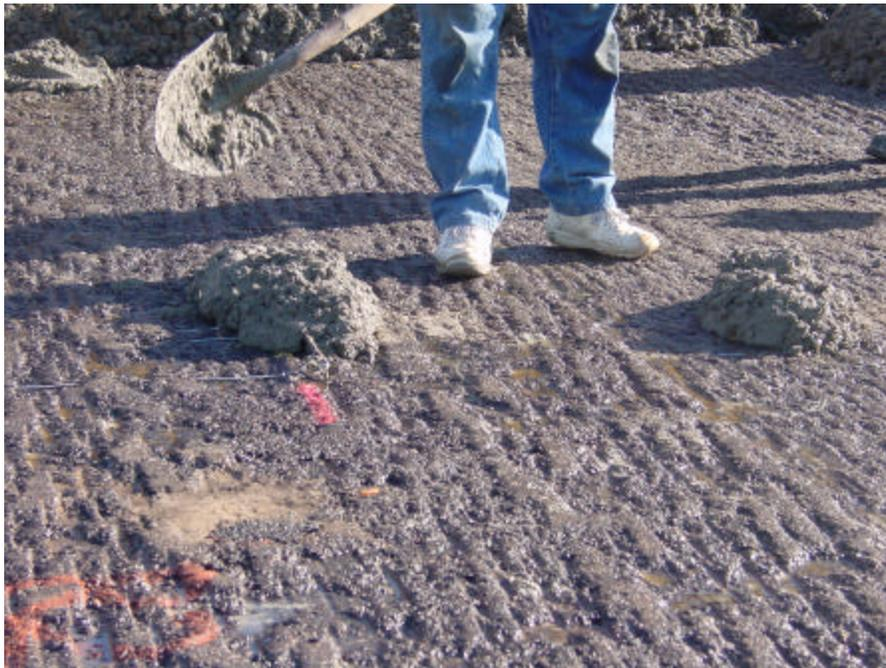
**Figure 34. Protection of Instrumentation Ahead of Concrete Paving**
