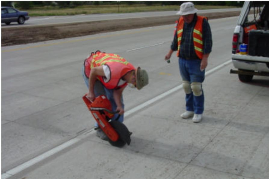
**Figure 24. Cutting Grooves Along Joints for Gage Cables**
