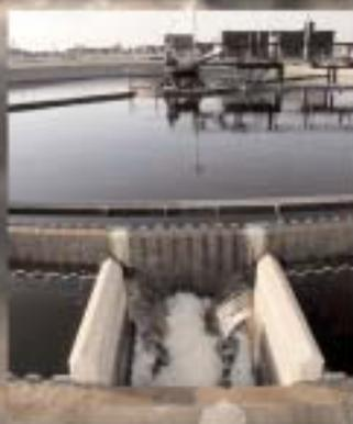
*Clockwise from top: The Metro Wastewater facility is the largest in Colorado. Raw sewage from municipalities across the Denver metro area enters the plant. The aeration pond, part of primary treatment, is sampled and monitored. The water moves to a secondary clarification pond. Chlorination ponds are the next to last stage before the effluent is discharged to the river.*
