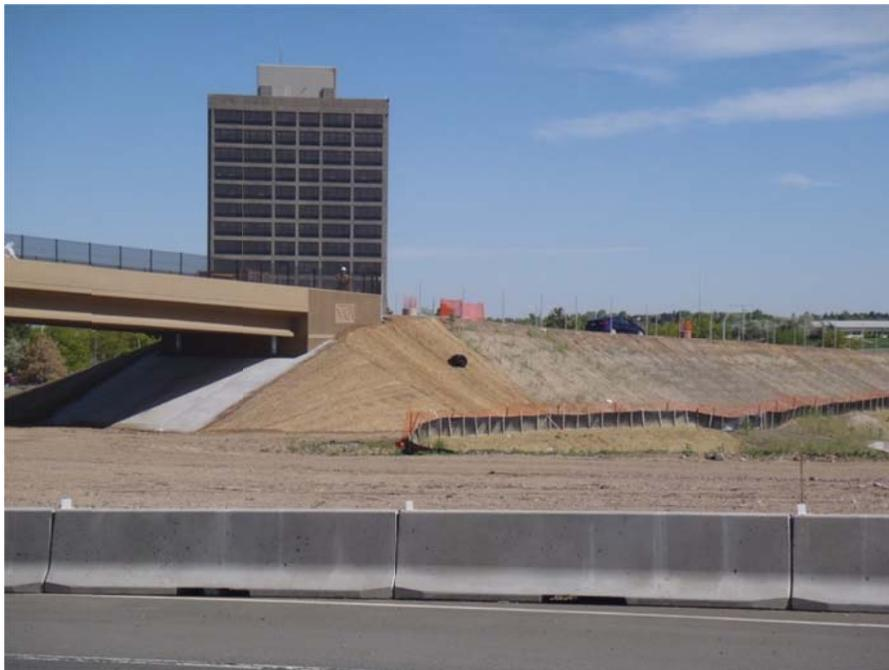
Figure 31. BMPs for RTD's light rail bridge construction in Lakewood over Highway 6.
